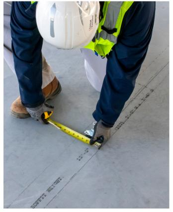
Above: The robot's markings are validated for accuracy.
