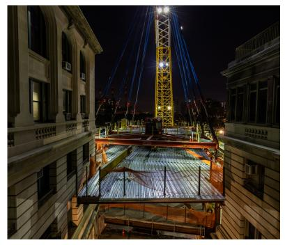
A module is carefully fit between two existing structures
