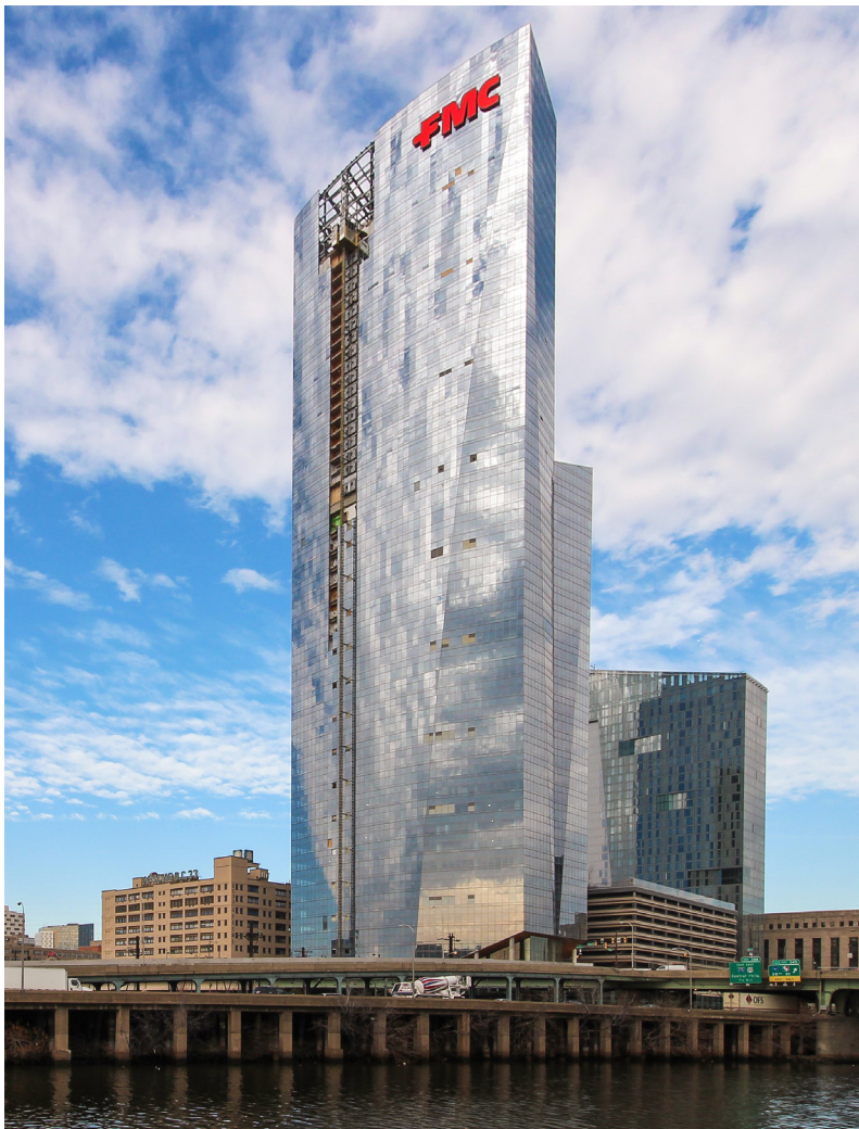
FMC Tower at Cira Centre South Philadelphia, Pennsylvania
