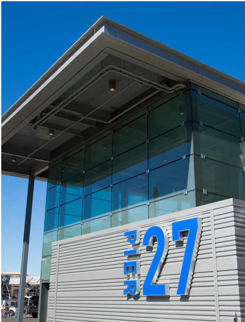
Pier 27 San Francisco, California
