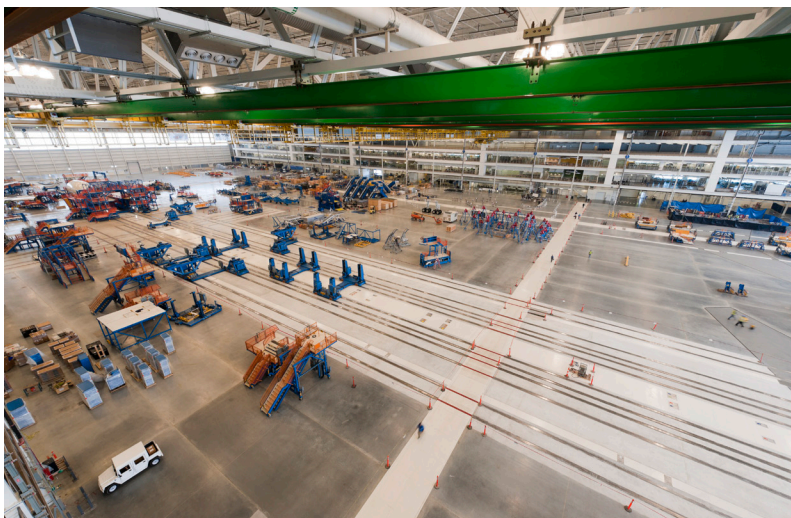
Boeing South Carolina 787 Final Assembly and Delivery Building North Charleston, South Carolina
